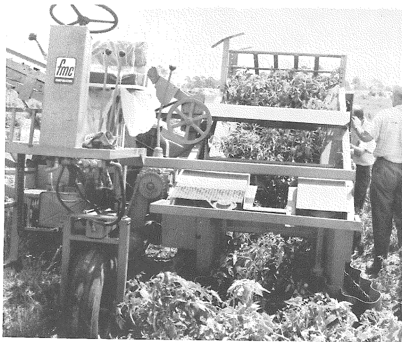
The machine in photo above was built to harvest tomatoes for the processing industry. It was found unsuitable for fresh market tomatoes. At right, W. W. Deen, Jr., of the Everglades Experiment Station, tests a principle which might work for handling fresh tomatoes.
