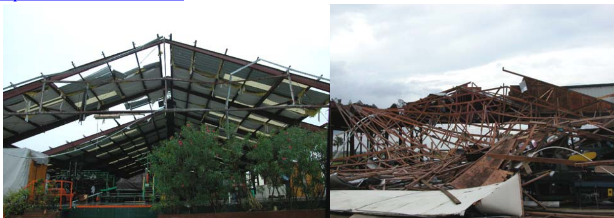
Fig. 3. Packinghouse Damage in the Indian River region from hurricanes Frances and Jeanne.
