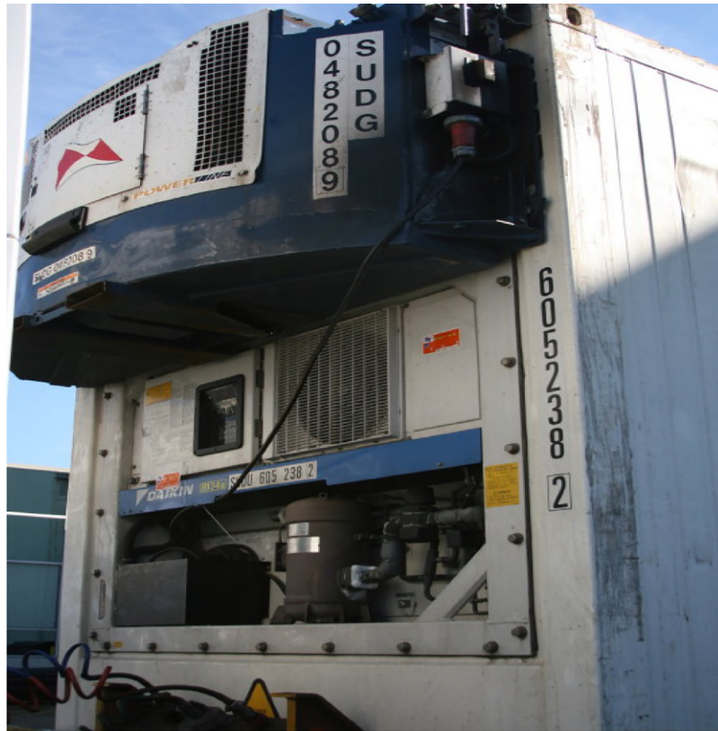
FIG. 18.5 Clip-on gen set mounted to a refrigerated container. Source: PEB Commodities, Inc.
