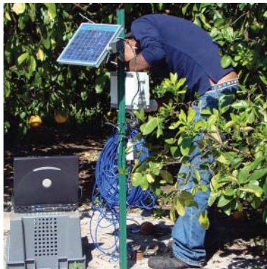
Sambhav works with photovoltaic station in a citrus grove
